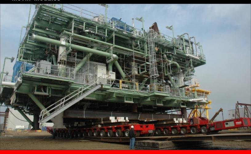
This job was a challenge due to the shallow water slip the barge was docked in. The barge height was 5' above the bulkhead so Berard engineers went to work designing and building a ramp system to move the 900 ton compressor onto the barge. Using 34 axle lines of Goldholfer transporters, the move was successfully completed on time and in a safe manner in only one day.
