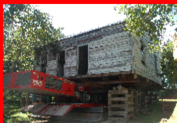
A combination of ramps and mats kept the load level for the final placement on the steep incline.
