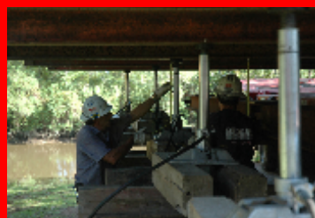
A combination of ramps and mats kept the load level for the final placement on the steep incline.
