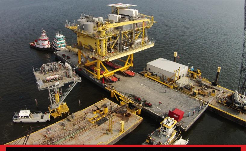
The final phase of the project was a history making event. Typically offshore platforms are installed onto their jacket structures by way of a derrick barge crane but due to the shallow water depth in Black Bay, a conventional installation proved nearly impossible. The engineers at Berard devised a plan to install the deck onto the jacket by lifting the deck with SPMTs then floating the barge and cargo between the jacket legs and using the SPMTs to lower the deck onto the jacket.
