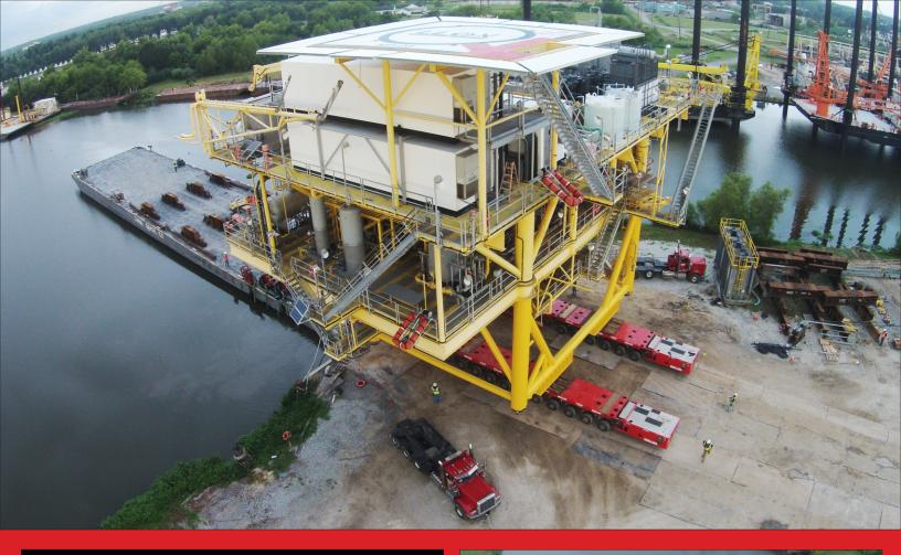
Once the refurbishment was complete, the deck and jacket were loaded onto a deck barge for water transport to the installation site. The key element was utilizing a narrow barge that would allow the deck legs to overhang for the installation phase. Having less width called for using a longer barge to compensate for the narrow width. Once on the barge, both cargo and Berard's SPMTs set sail to the installation site at Main Pass 23 in Black Bay near the Gulf of Mexico.
