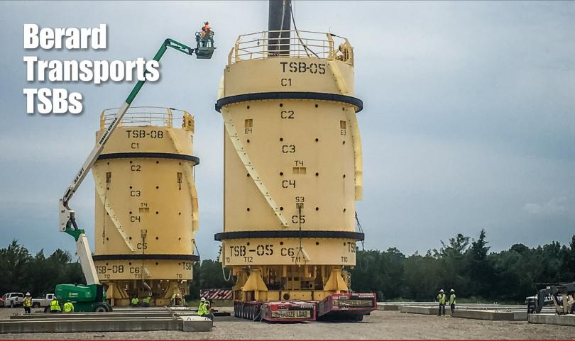
Job Specs Weight: 134 Tons Dimensions: 31' D x 54' H
